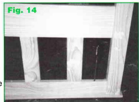
Do a dry run for each capping piece and then glue and screw them in place (**Fig. 14**).
